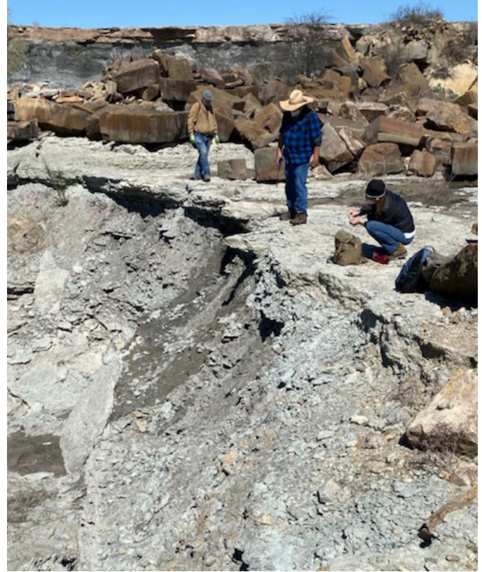
Exploring the spillway at Lake Brownwood Photo by Jamie Shelton
